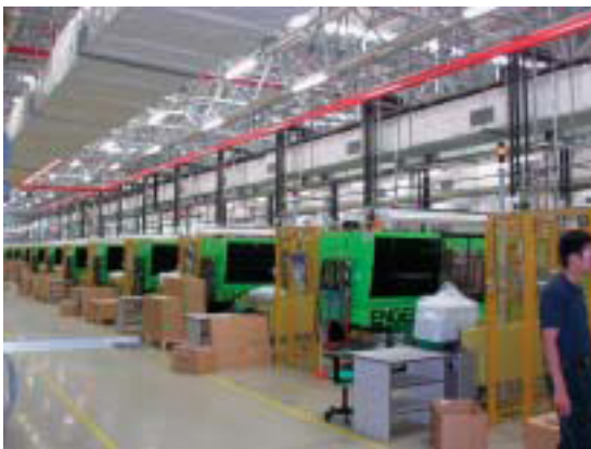
Overhead air conditioning ductwork in a factory.
