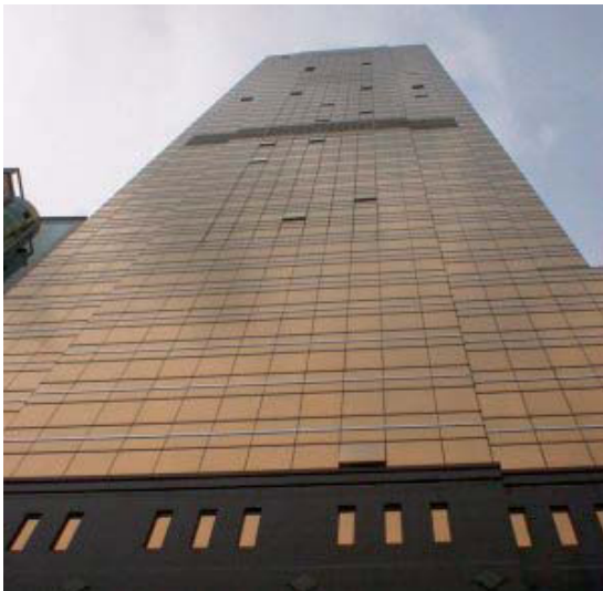
Air conditioning is an important element in high rise office buildings (Guangzhou, China).
