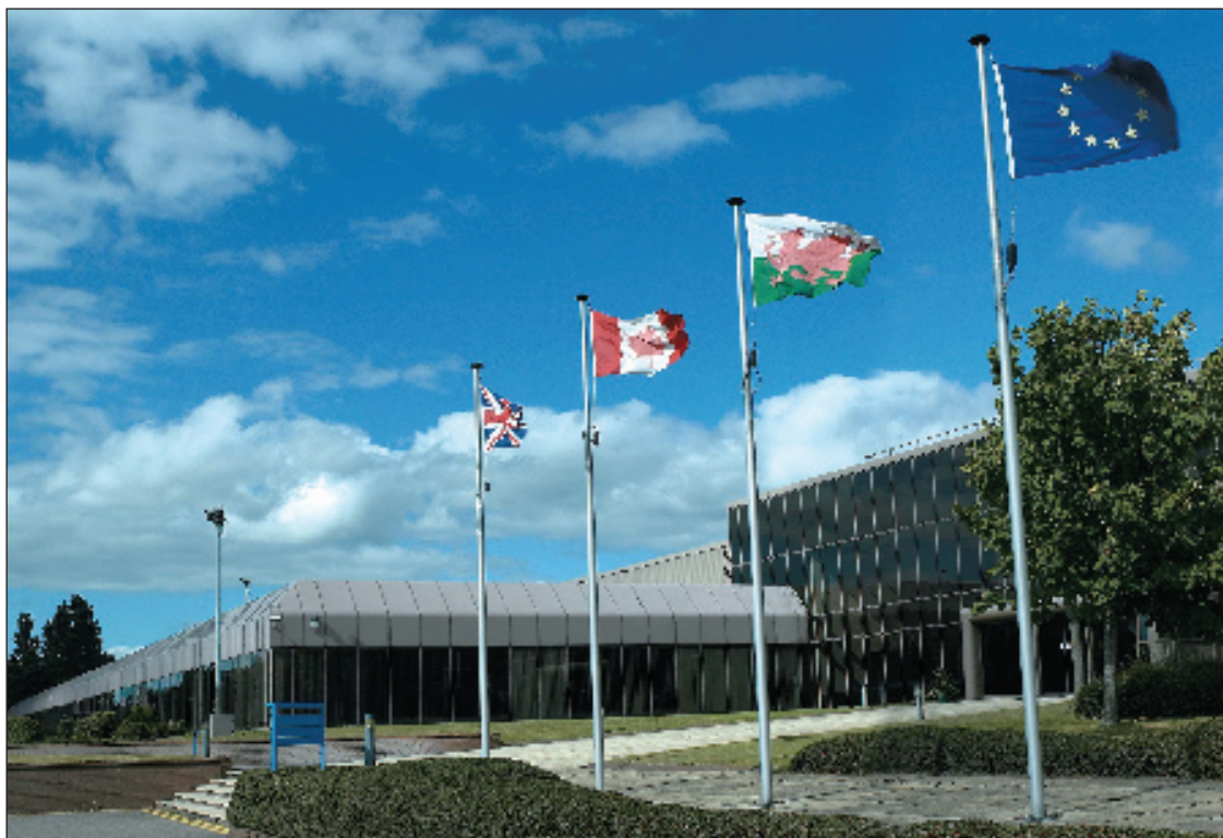
Two ABB standard drives for HVAC have reduced energy costs from £180 to just £50 a week, giving an annual saving of over £6,000.
