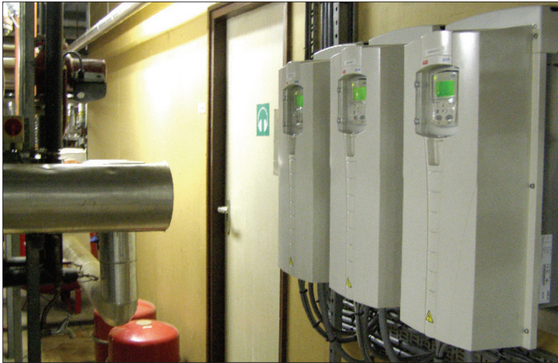
ABB standard drives for HVAC helped to reduce energy consumption by at least 10%.
